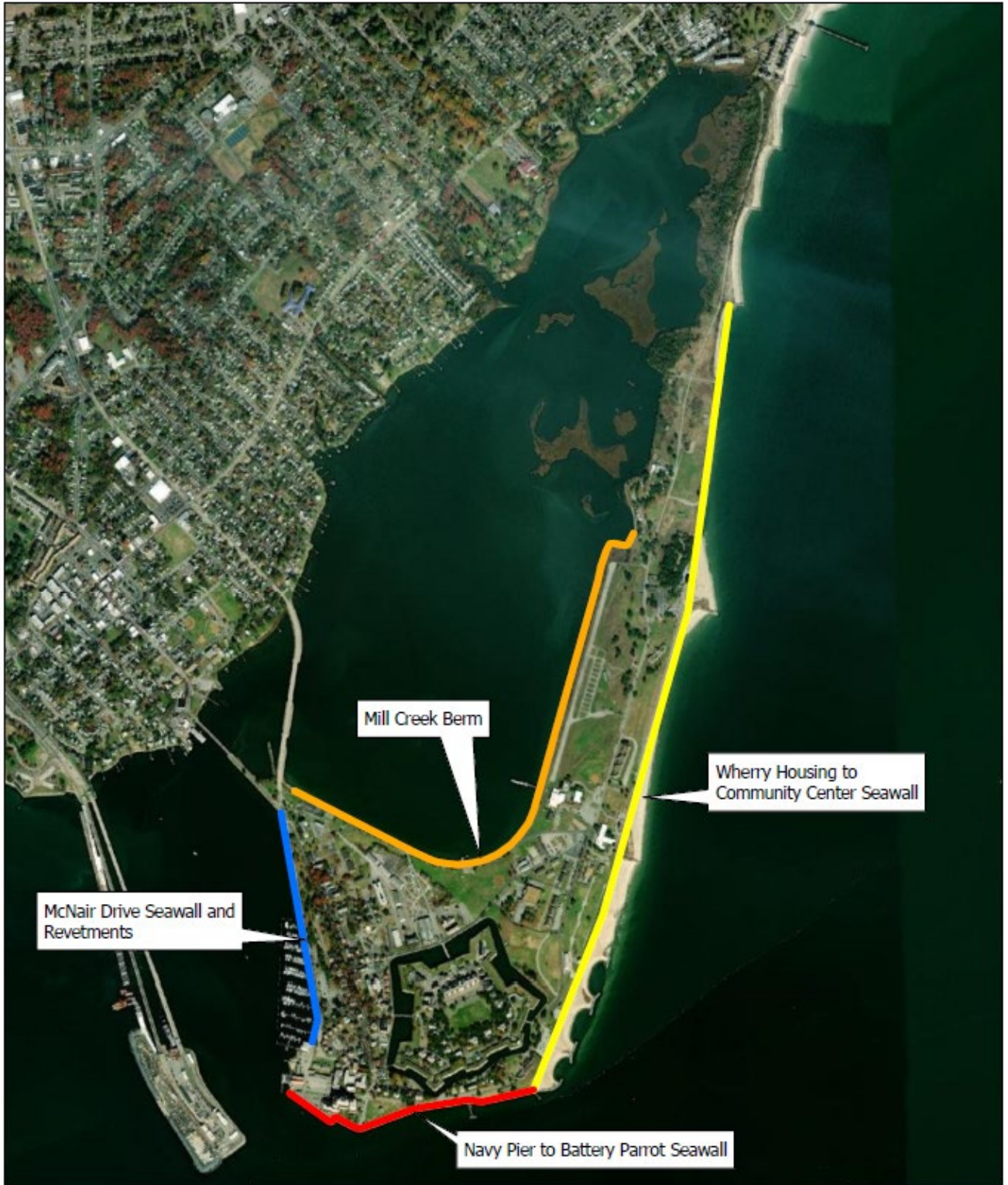
Figure 9: Fort Monroe Seawalls and Berm
