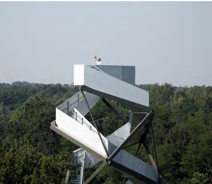
Tower at the Mur River, Austria
