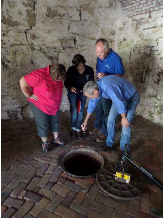
Figure 3 & 5 Casemate Cultural Resources Manager, Veronica Gallardo, leads the Historic Structures Report team on an examination of the scarp wall and a manhole in the postern gate.
