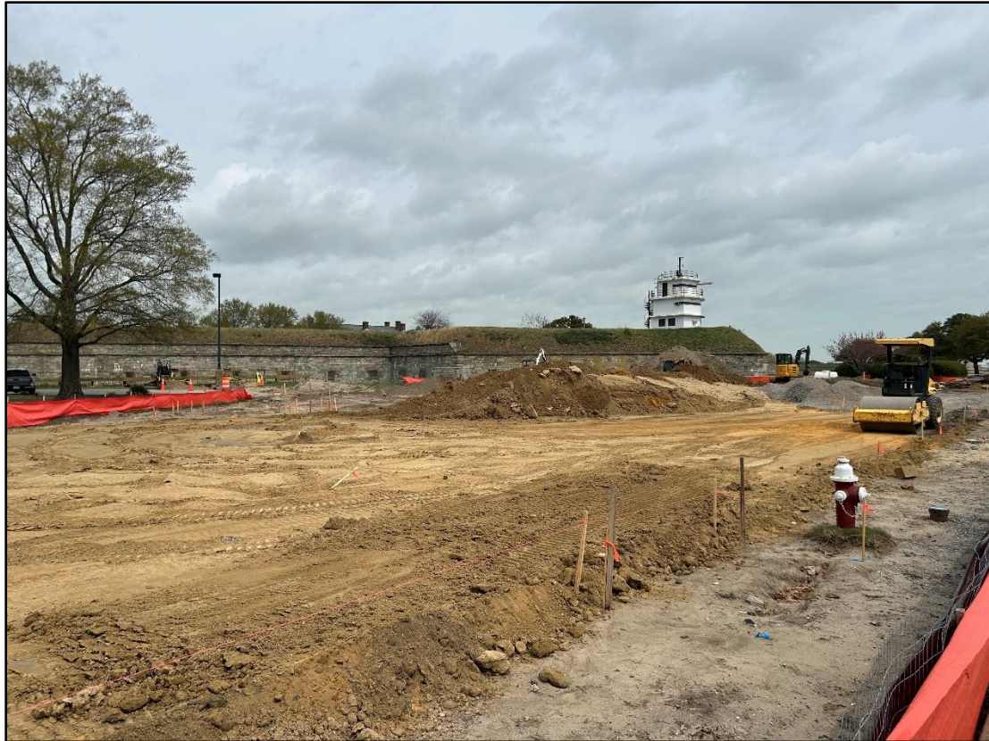
Showing Zone F looking NE across location of new parking area
