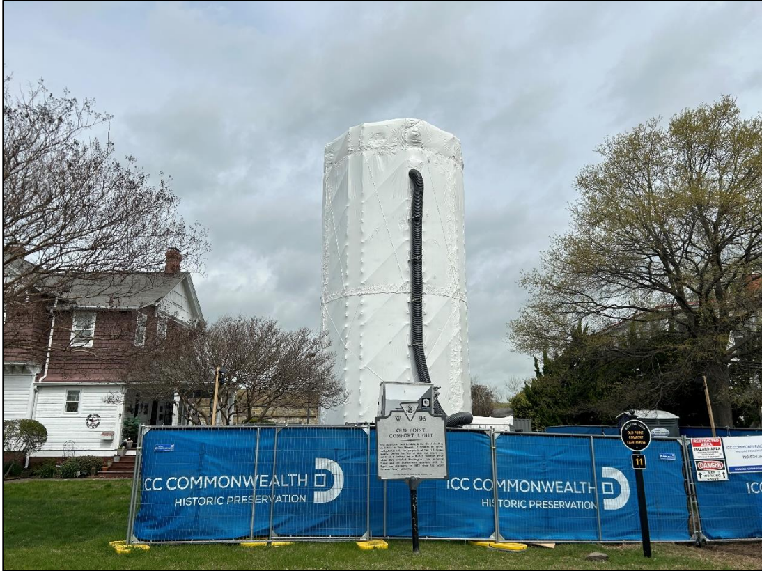
Image showing Scaffolding and containment at the Old Point Comfort Lighthouse
