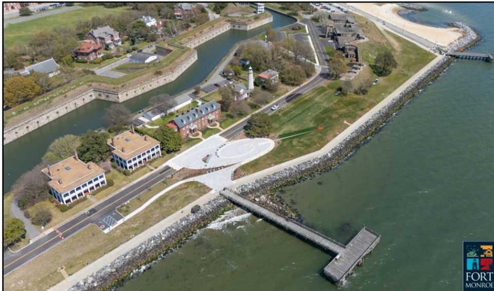
Image showing Zone A of the ALM Plaza Site as of April 1, 2026
