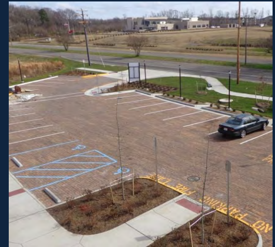
Permeable Paving, Chesapeake, VA
