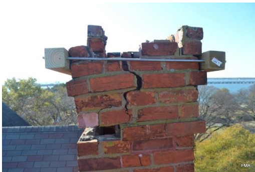
Chimney struck by boom lift, initial stabilization
