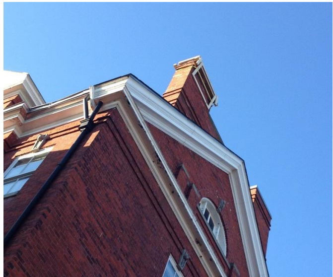
Chimney struck by boom lift, current
