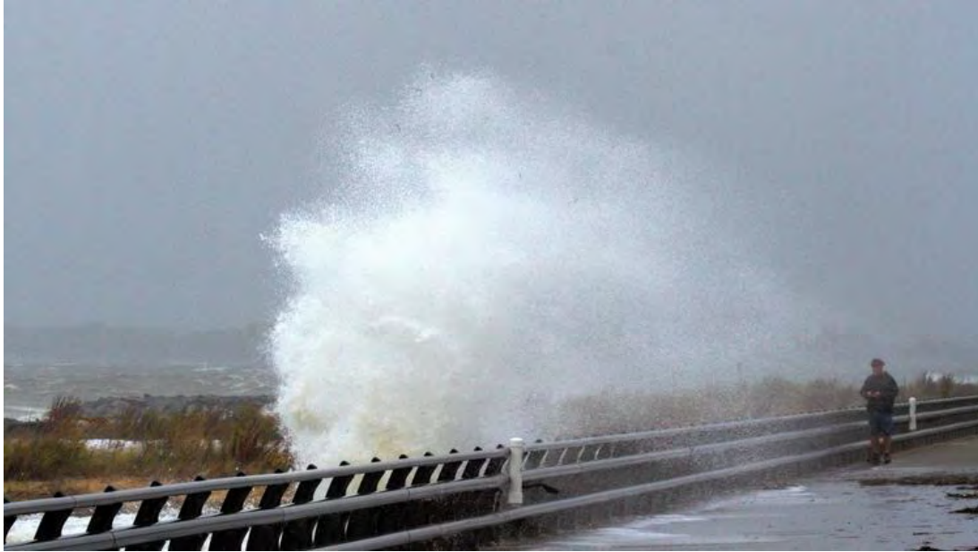
Storm driven surf pound everything its path in this view of the seawall at Ft Monroe on Sunday, Oct. 4, 2015. (Adrin Snider / Daily Press)
